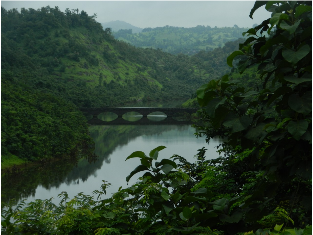
Figure 26: Submergence of Middle Vaitarna Dam Photo: SANDRP
