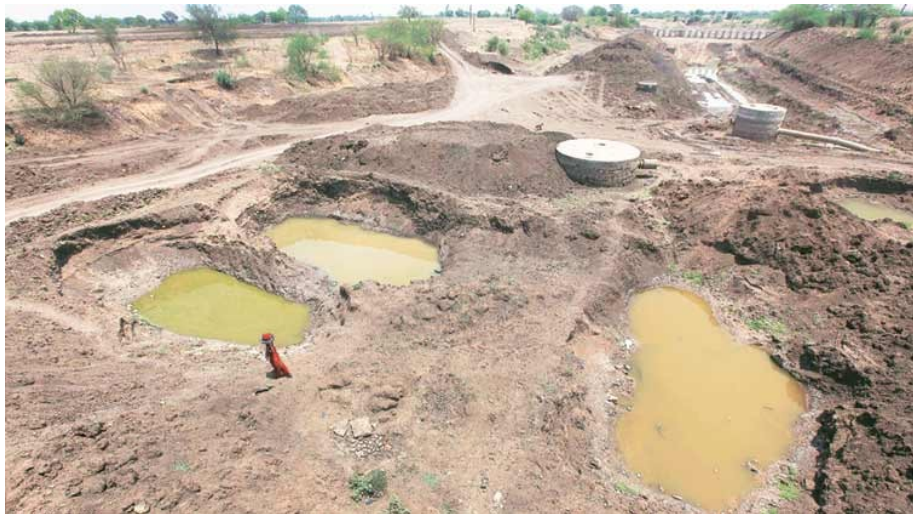
Figure 16: Unscientific deepened and widening of Manjra River in name of rejuvenation Photo: Indian Express
